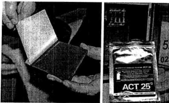
Photo 29258d-22 and 25: Installation of PiroStiker AST-25
