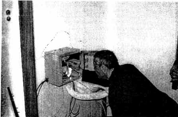
Photo 29258d-8: Ignition of the telephone cable hanged in the cabinet. Burning of the cable within the cabinet without PiroStiker last approx.1 minute.
